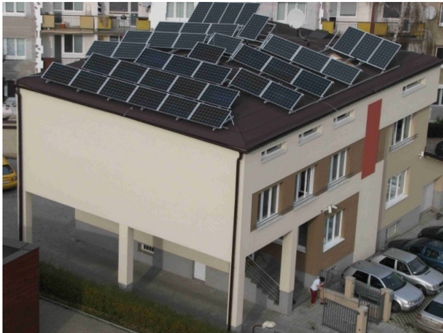
Fig. 1. Installed photovoltaic system
