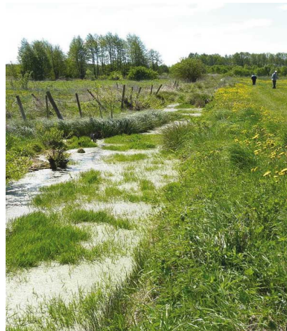
Fig. 4. Degradation of land improvement systems
