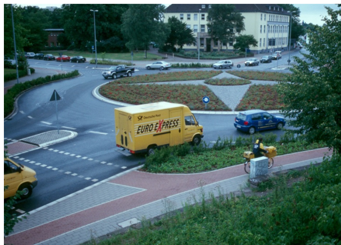
Fig. 7. Typical German compact semi-two-lane roundabout; Oberhausen (source: Werner Brilon)
